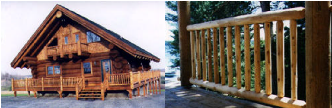
Figure 2 Round-wood railings and posts
