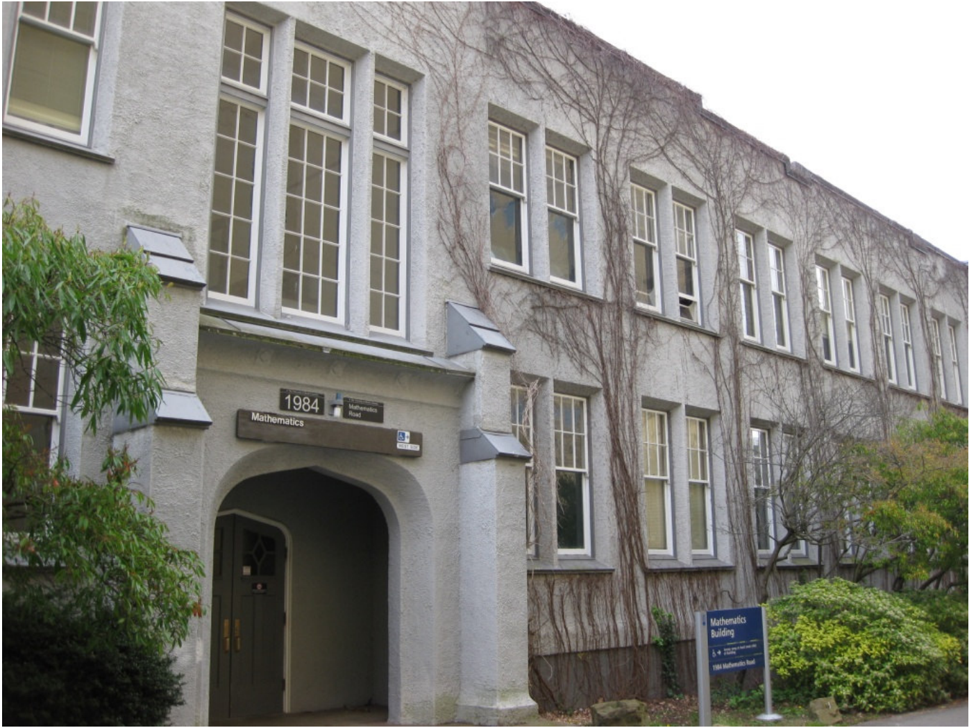
Figure 1 - Front Entrance of the Math Building
