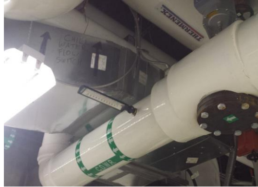
Figure 4: ESB: Thermenex header, with chilled water connection
