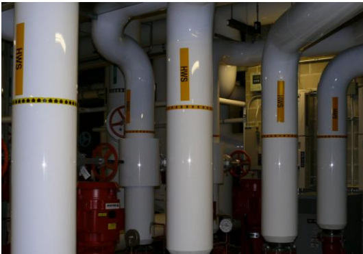
Figure 5: PSB: four pumps and headers, connected to four boilers indicating redundancies in hot water supply
