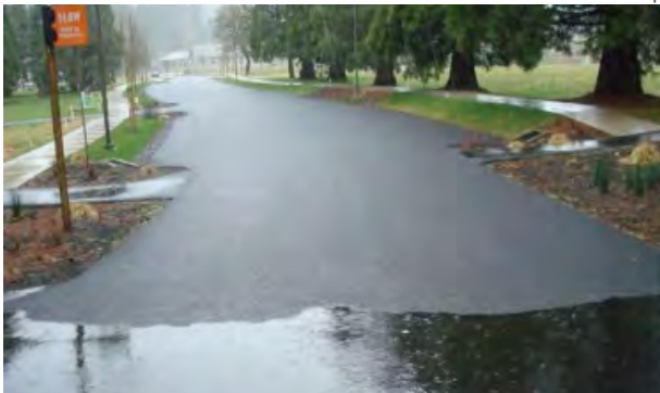
Figure 38 Pervious paving used in Pringle Creek allows water to percolate through. Image from http://www.ewashtenaw.org
