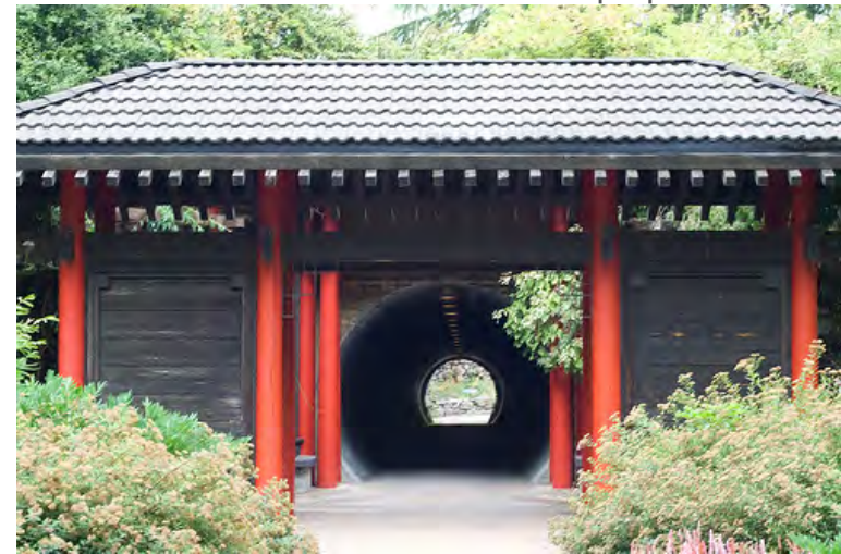
Figure 35. This is an existing tunnel in the UBC botanical garden.
