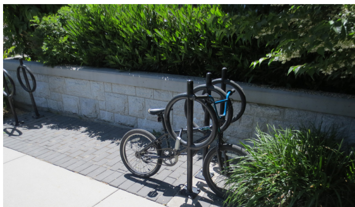
Figure 32: Ring and post locks also provide a stable and secure rack. Other posts can be retrofitted with rings to create them.
