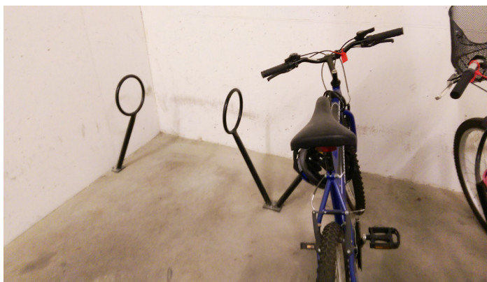
Figure 31: V-racks are difficult to balance bicycles against and can't support small and long bicycles without kickstands.
