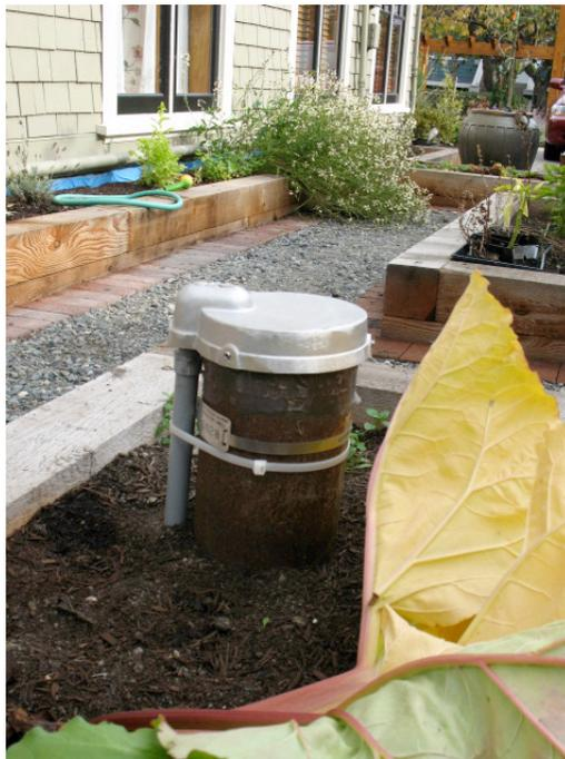
**Figure 14 - Geothermal well head (disguised by raised vegetable bed in south side garden)**
