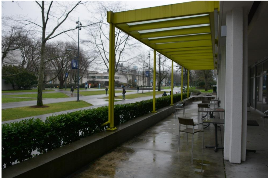
Figure 24: Covered patio café outside the Henry Angus Building, overlooking Martha Piper Plaza, UBC Point Grey Campus, Vancouver.
