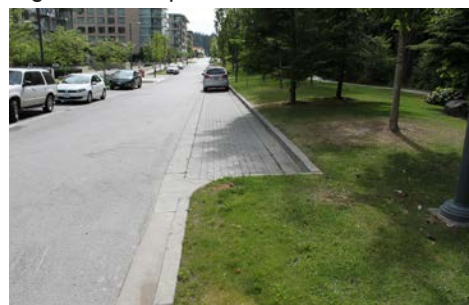
Figure 5.9 On-street parking with permeable paving
