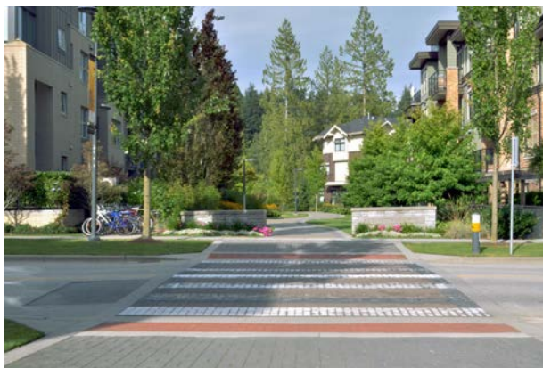
Figure 3.9 Elevated crosswalk on Wesbrook Mall
