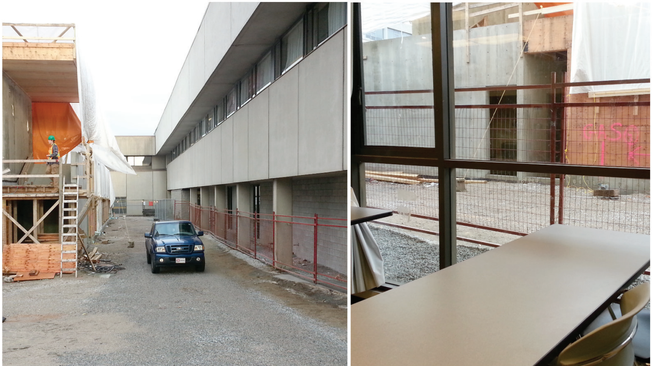
Figure 4. CEME classroom adjacent to construction site.
