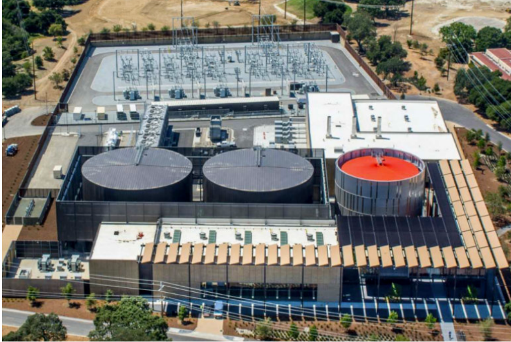
Figure 10 – Stanford energy facility with hot water storage in red Source: University, S. & Golden, M. (2019, May 07)
