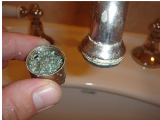
Figure 3: Accumulated Silt Inside an Aerator
