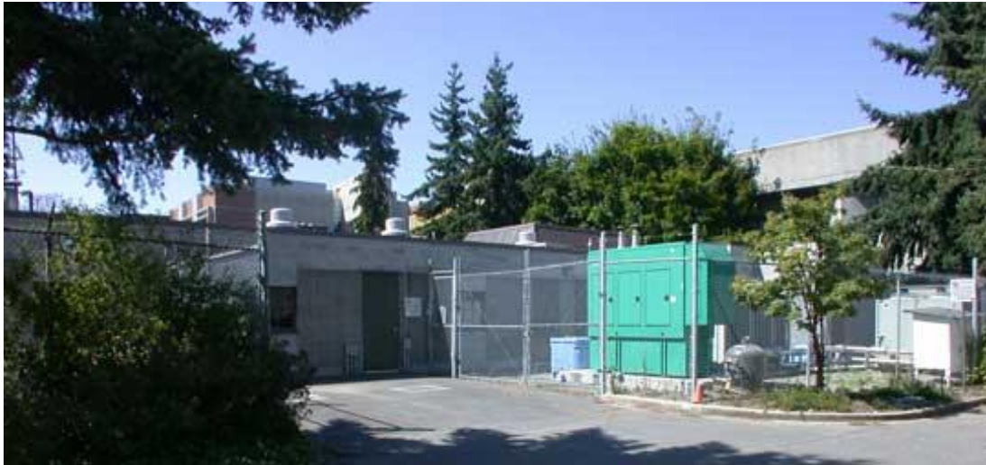
Figure 8: Outdoor Aquatic Facility, University of Victoria, Saanich, BC
