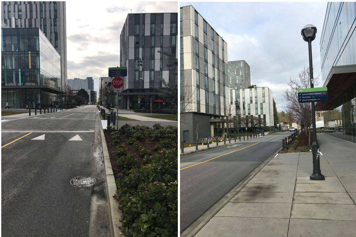
Figure 7. Inconsistent signage locations at the West Mall intersection.
