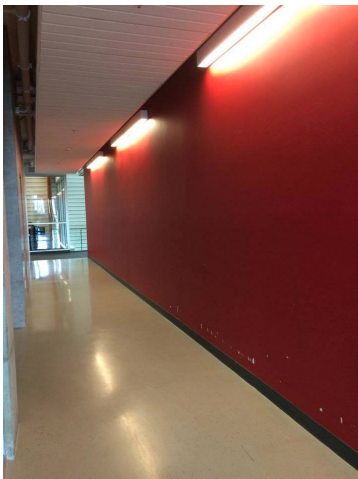
Figure10: Wall in north corridor
