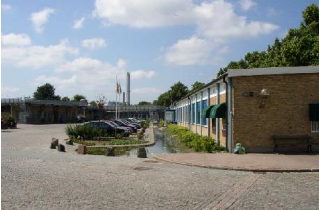
Figure 5 - Storm water collection ditch (Villarreal, Semadeni-Davies, & Bengtsson, 2004)
