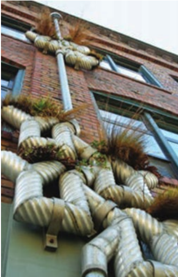
Figure #22 Roof runoff at 81 Vine is directed to these candelabra downspouts, whose playful forms evapotranspire some rainwater and oxygenate the rest (Echols & Pennypacker, 2015)
