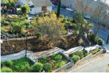
Figure #21 Tiered infiltration basins step down the slope, with any overflow at the bottom directed to the city sewer system (Echols & Pennypacker, 2015)
