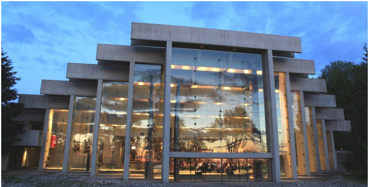
Figure 1. MOA building in UBC. 15m high windows present on the north end of the Museum of Anthropology, facing the water and trees.
