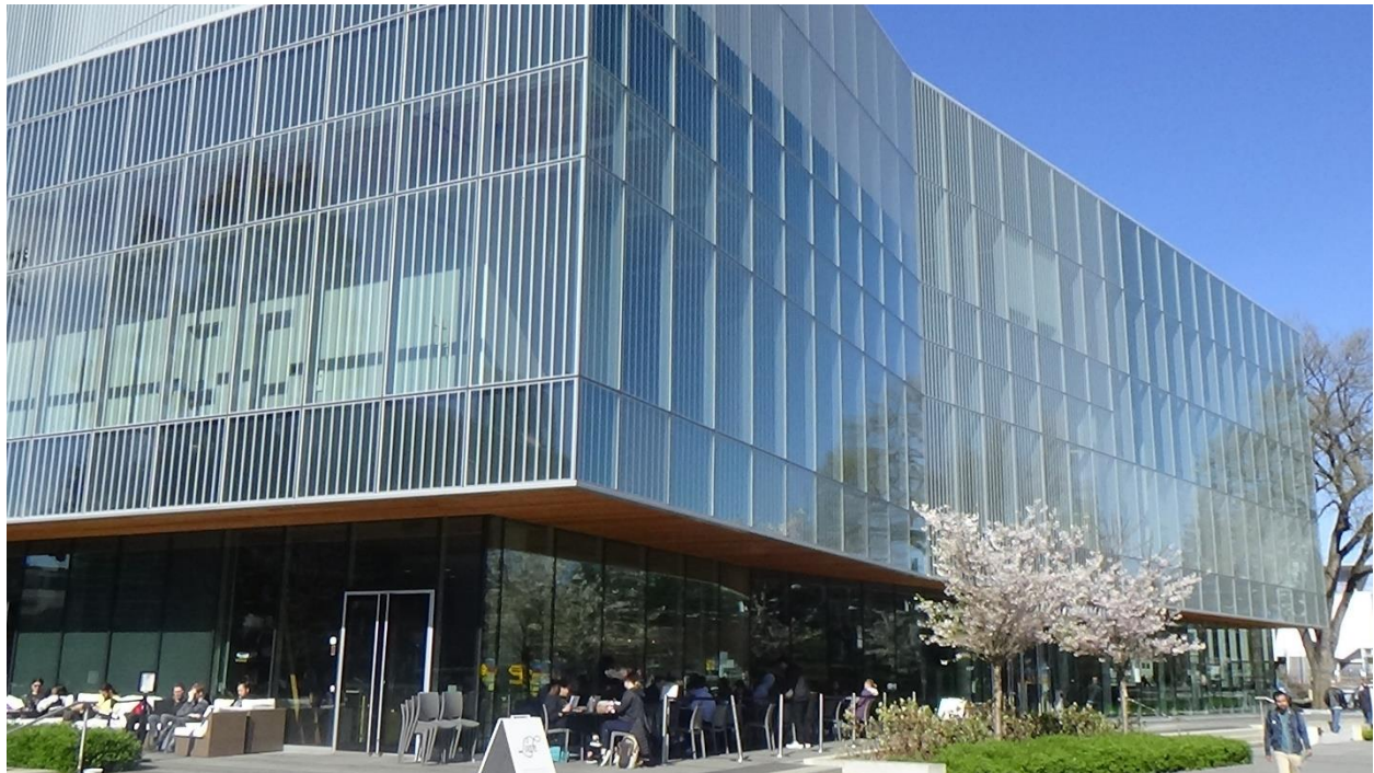
Figure 5. Robert H Lee Alumni Centre. The center has vertical white stripes on the large window, which is effective preventing strikes of birds.
