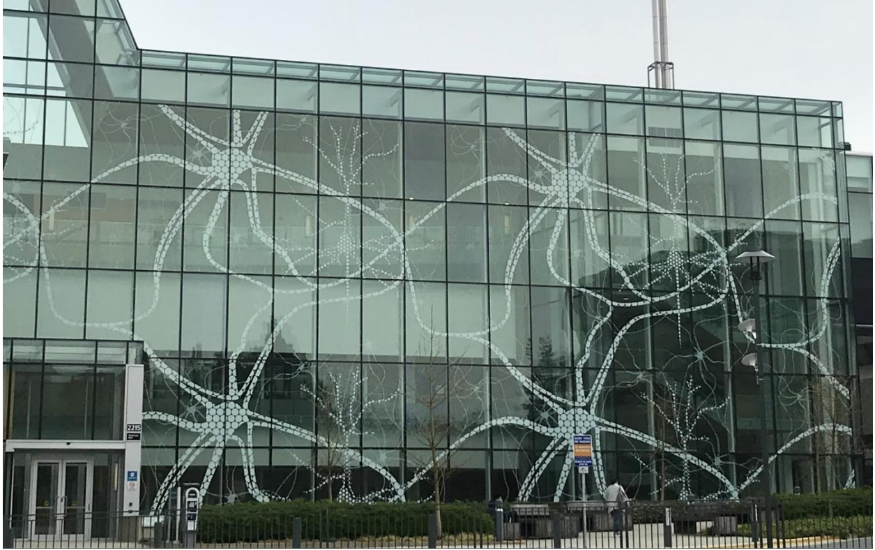
Figure 9. UBC Hospital. The metallic pattern could help increase the visibility of the glass wall. But the efficiency is unknown since it is not following the 2 x 4 rule.
