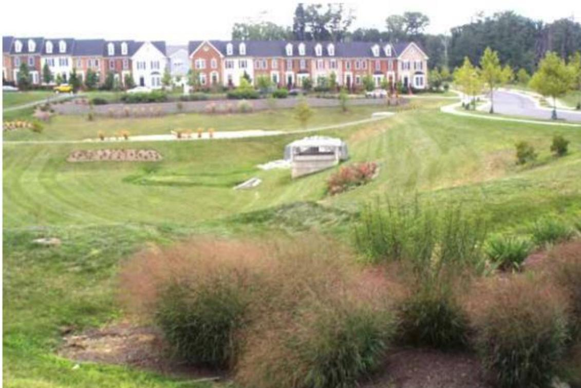
*Figure 10 Example of a Dry Pond*
