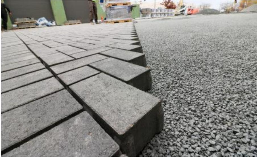
*Figure 4 Example of Partial Installation of Pervious Pavers*
