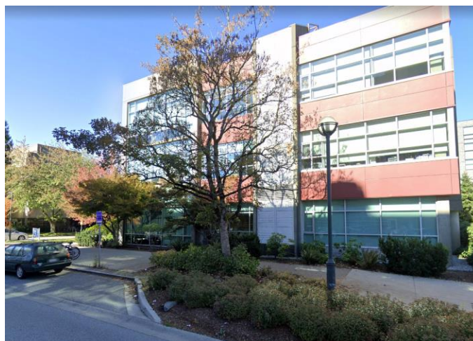
Figure 8: Street view of Gerald McGavin Building along Agronomy Rd (Captured on Google Maps)
