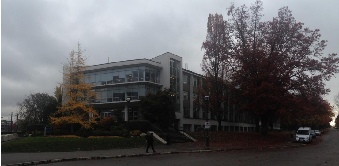
Figure 2 the Wesbrook Building
