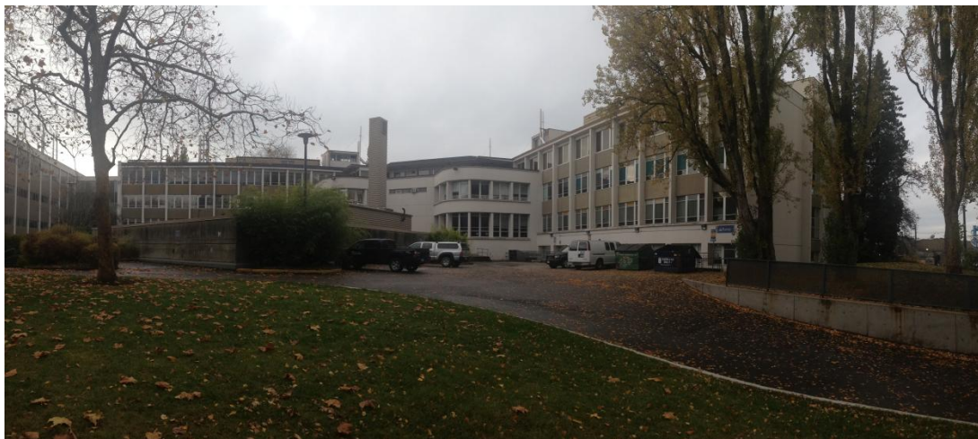
Figure 3 the Wesbrook Building
