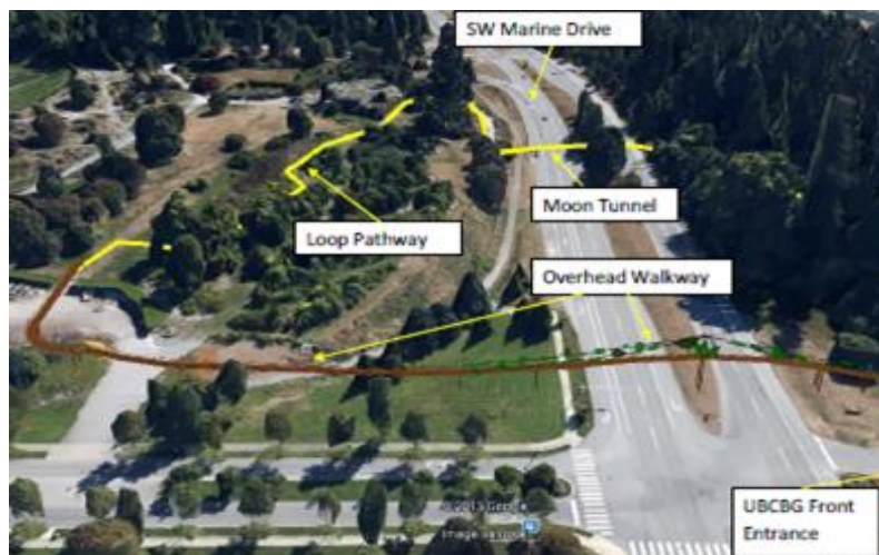
Figure 10: View of Overhead Walkway Looking South.
