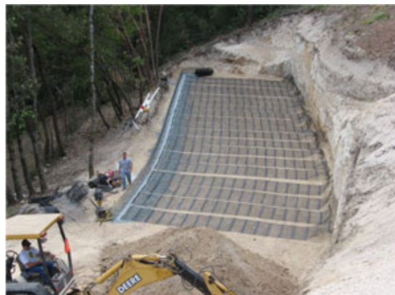
Figure 20: Mechanically stabilized earth (MSE) wall ( williamsae.com ).
