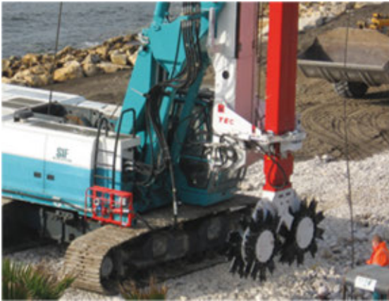
Figure 23: Soil mixing head on modified excavator (enr.construction.com).
