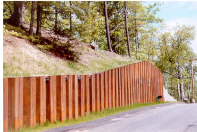
Figure 24: Sheet pile wall (kshijita.com).
