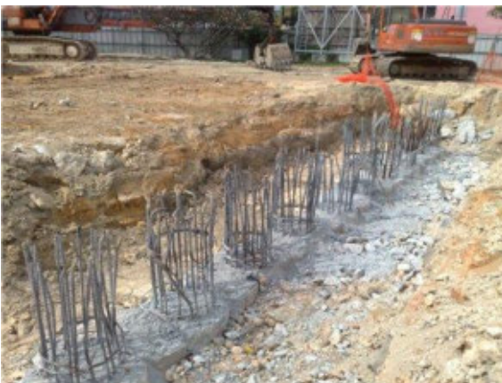
Figure 19: Secant pile wall ( foundation-alliance.com ).
