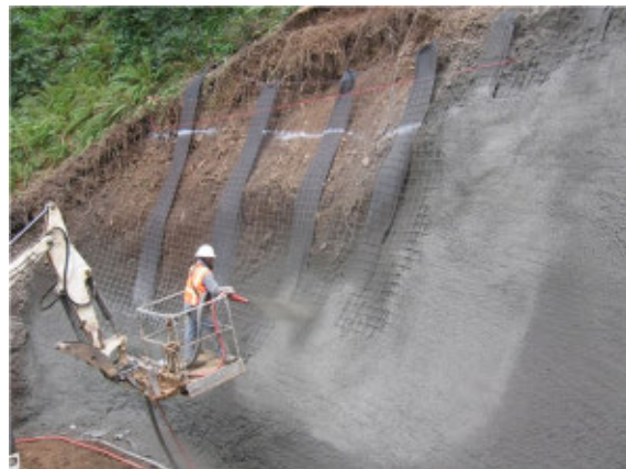
Figure 22: Shotcrete shoring ( plisystems.com ).
