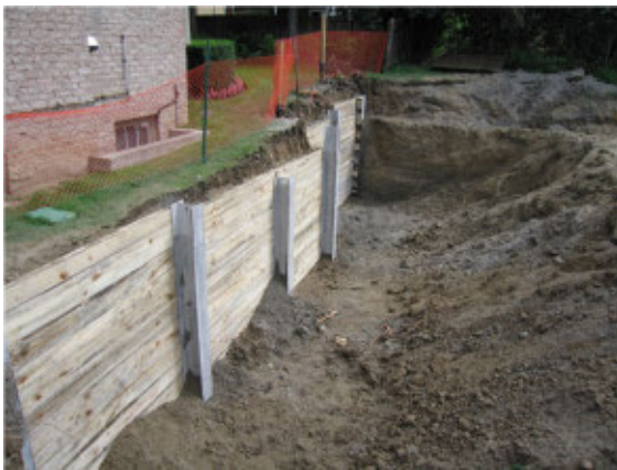
Figure 21: Soldier piles and lagging ( hcgroupp.ca ).
