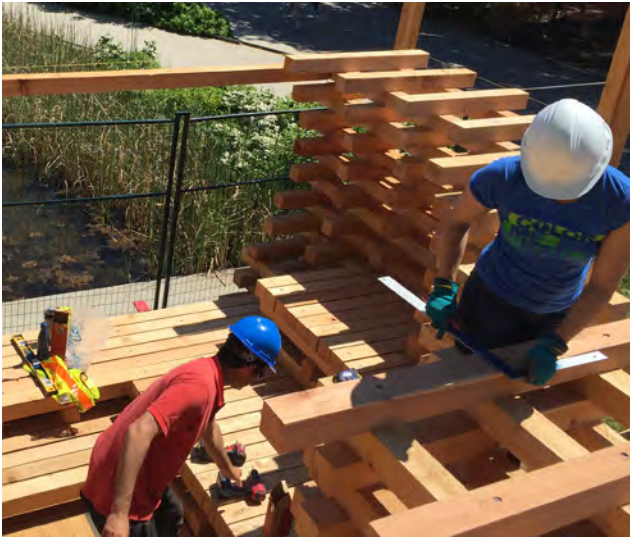
Clockwise from top left: construction of timber sub-frame; sorting shoring timbers, securing decking; corbelling over entrance; ensuring shoring is square.
