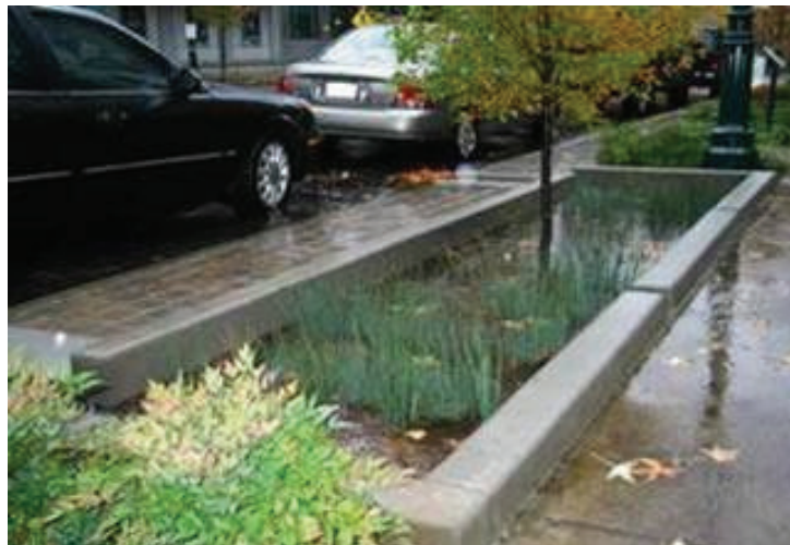
Figure 10. Bioretention Trees Example
