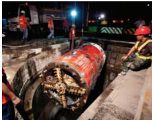
Figure 13. MTBM being lowered into access shaft (Source: Microtunnelling Systems)
