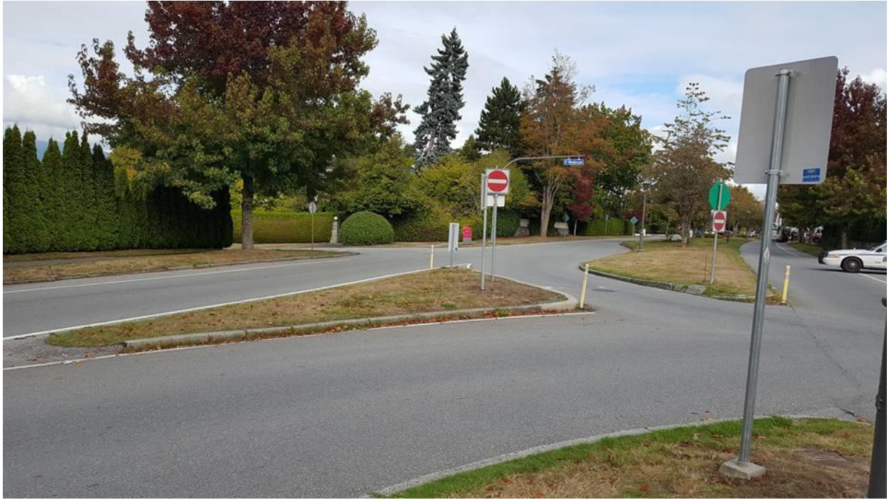
Figure 29 Photo of Site Facing East 1
