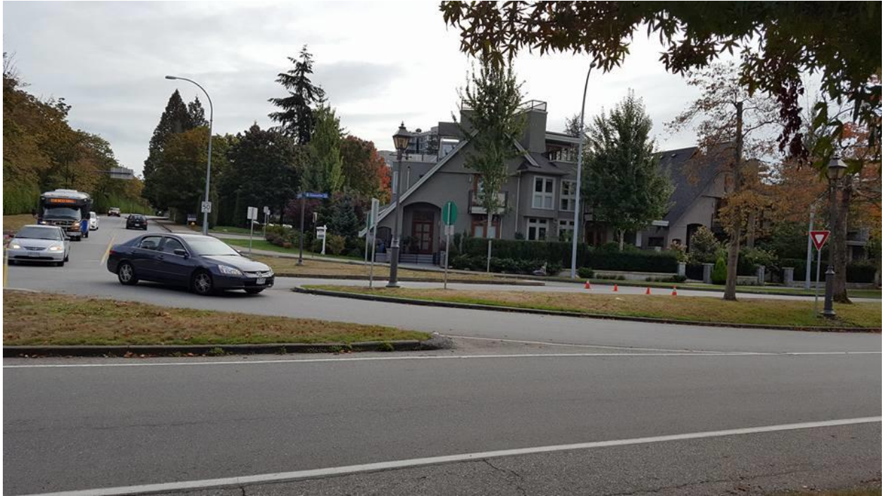
Figure 27 Photo of Site Facing South 3
