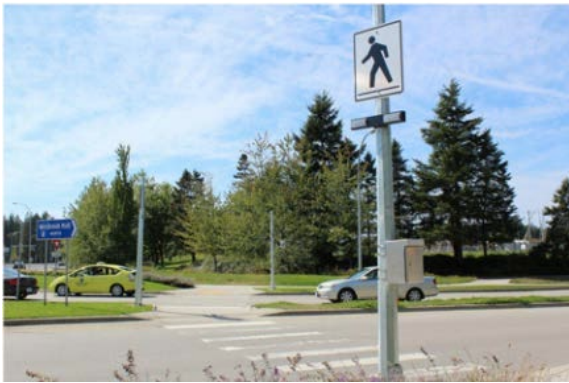
Figure 4 Short Pedestrian Crossings (Google earth)
