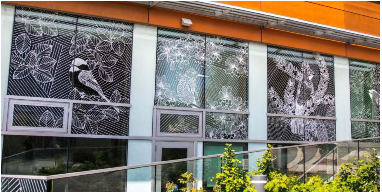
Bird-friendly window design at the Centre for Interactive Research on Sustainability (CIRS) on the University of British Columbia Vancouver campus.
