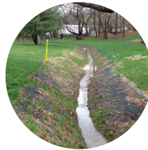
A shallow ditch to help with rainwater drainage
