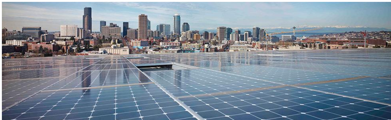
Figure 9 The Bullitt Center has 575 solar panels on the roof, creating a 14,000 square-foot array to generate electricity
