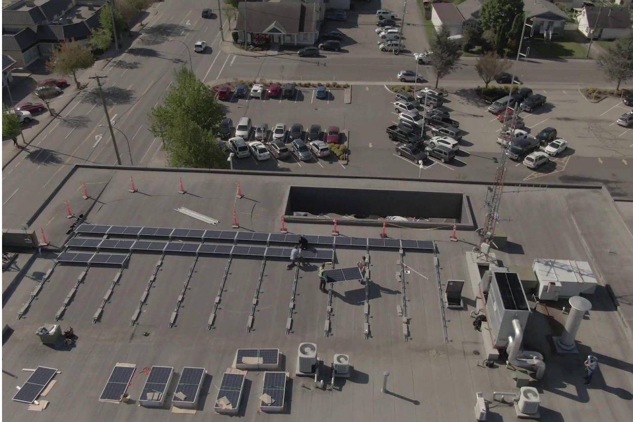
Figure 8 The installation of solar panels on the building's rooftop in downtown Chilliwack
