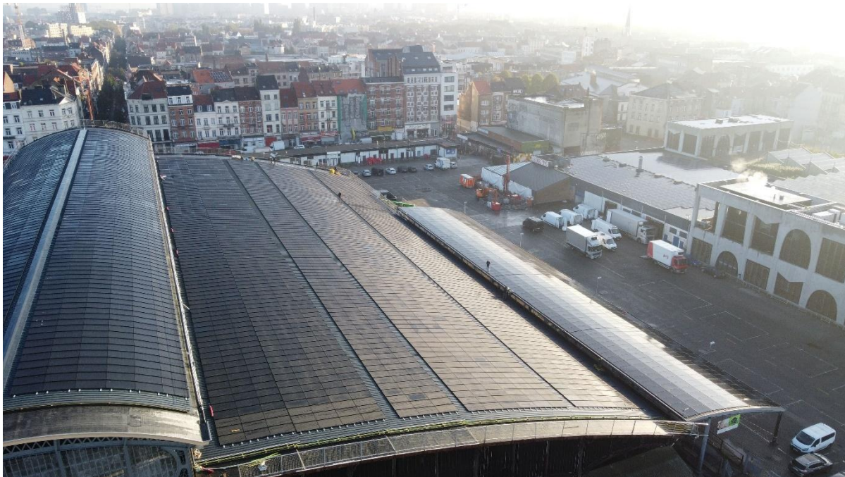
Figure 13 The SolarMarket – the first BIPV installation on heritage building in Brussels
