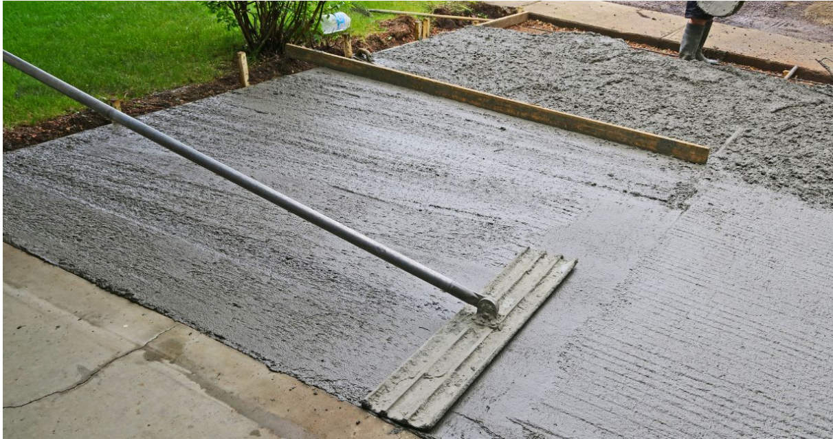
Figure 8. Sidewalk Concrete Construction (Image source: https://todayshomeowner.com/driveway/guides/concrete-thickness-for-driveway/ )
