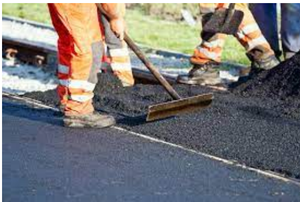
Figure 9. Asphalt Sidewalk Construction (Image credit from: https://www.builderspace.com/why-are-roads-made-of-asphalt-and-not-concrete )
