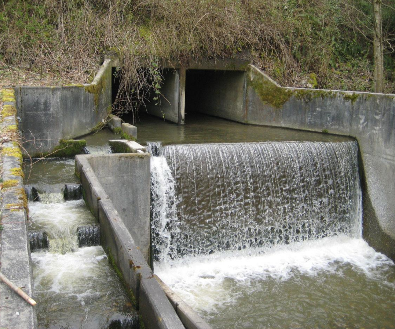
Anderson Creek fish ladder, Washington State Dept of Transportation, via Flickr
