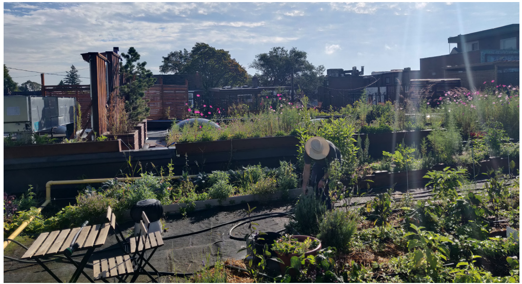
The Carrot Green Roof & Garden, Toronto, Canada, photograph by Ryan Godfrey.
