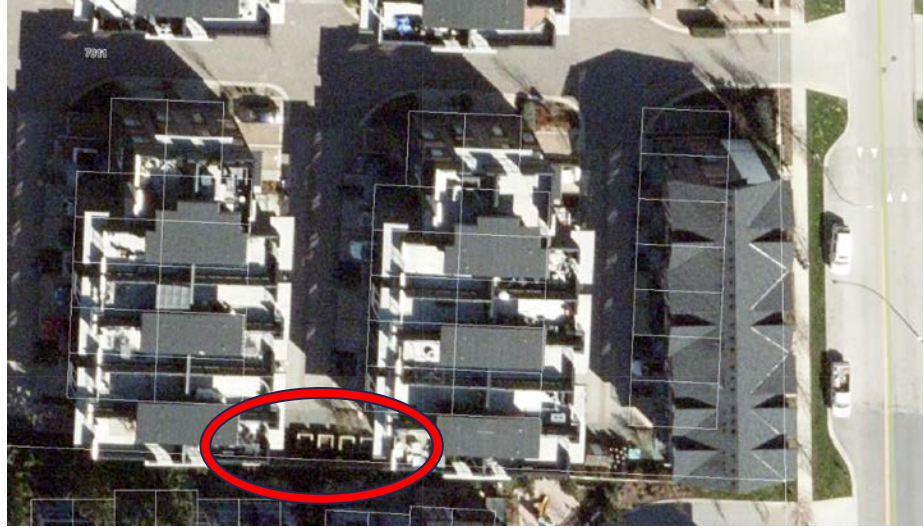
Figure 22. An Aerial View of The Exchange Apartment Complex with Garden Plots in a Red Circle (Image by the Township of Langley)
