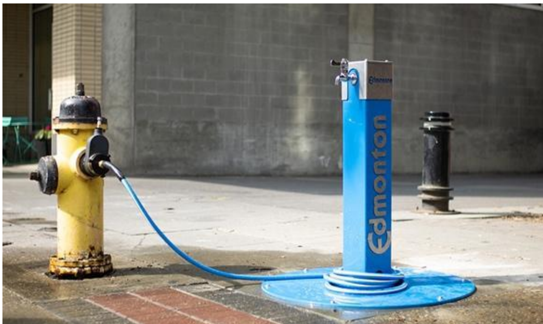
Figure 61: A fire hydrant that connects to a drinking water station in Edmonton, AB
