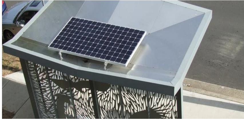
Figure 67: Solar power on the CAPS shelter in Sydney, Australia
