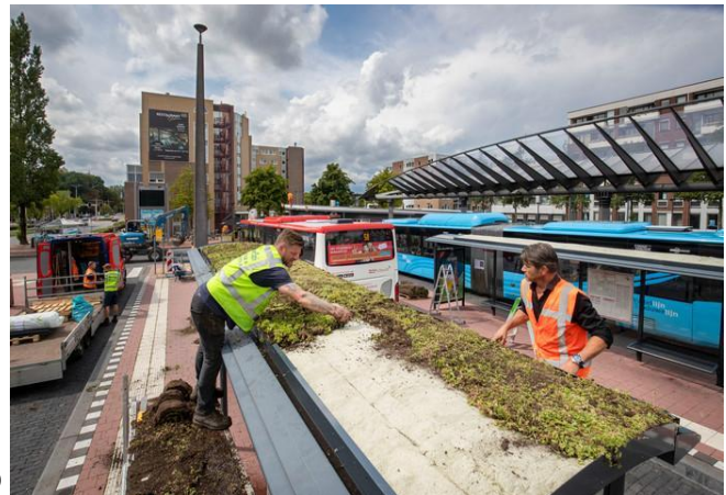
Figures 62, 63: Green roof installed on a transit shelter in Utrecht, The Netherlands
