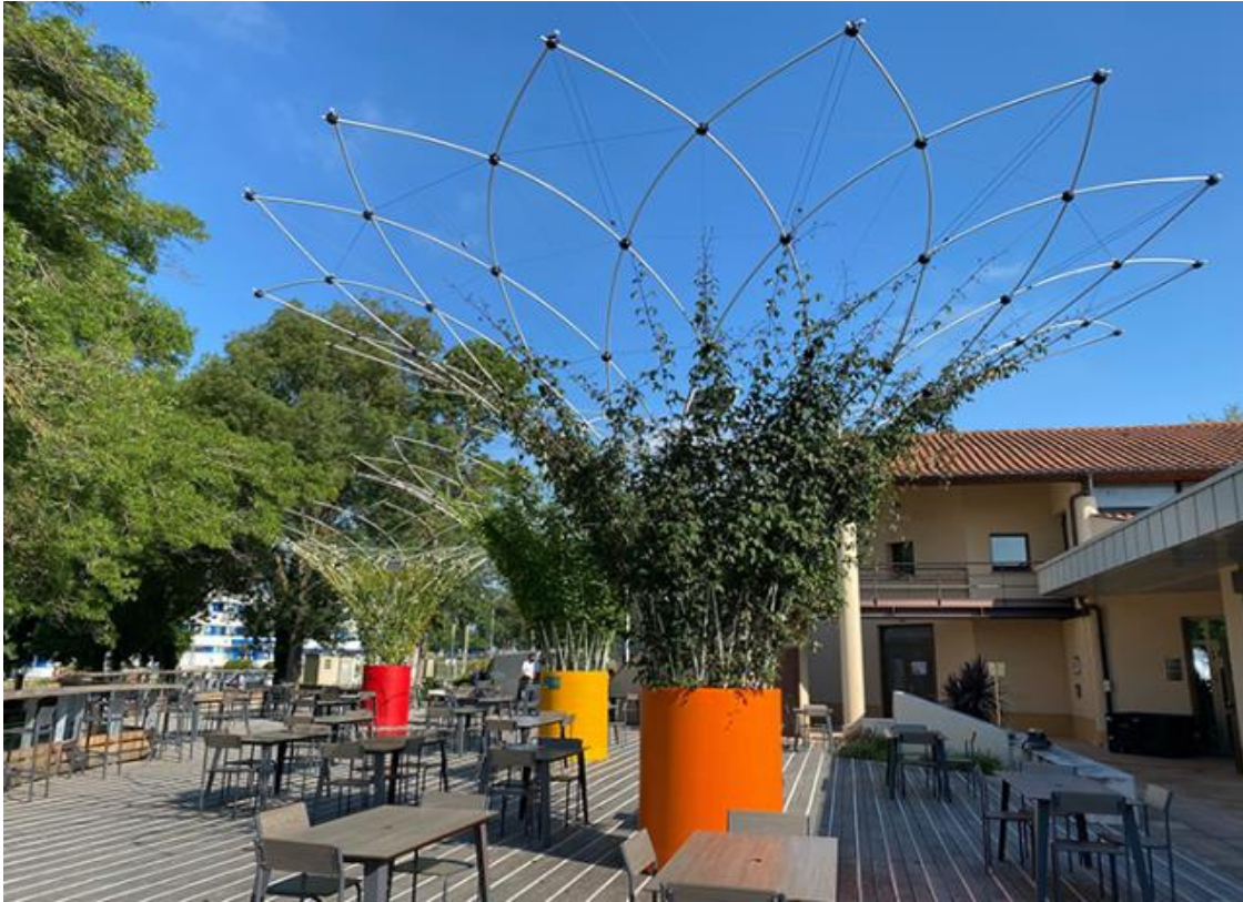
Figure 70: the Canopee creates a freestanding shade canopy with incorporated irrigation
