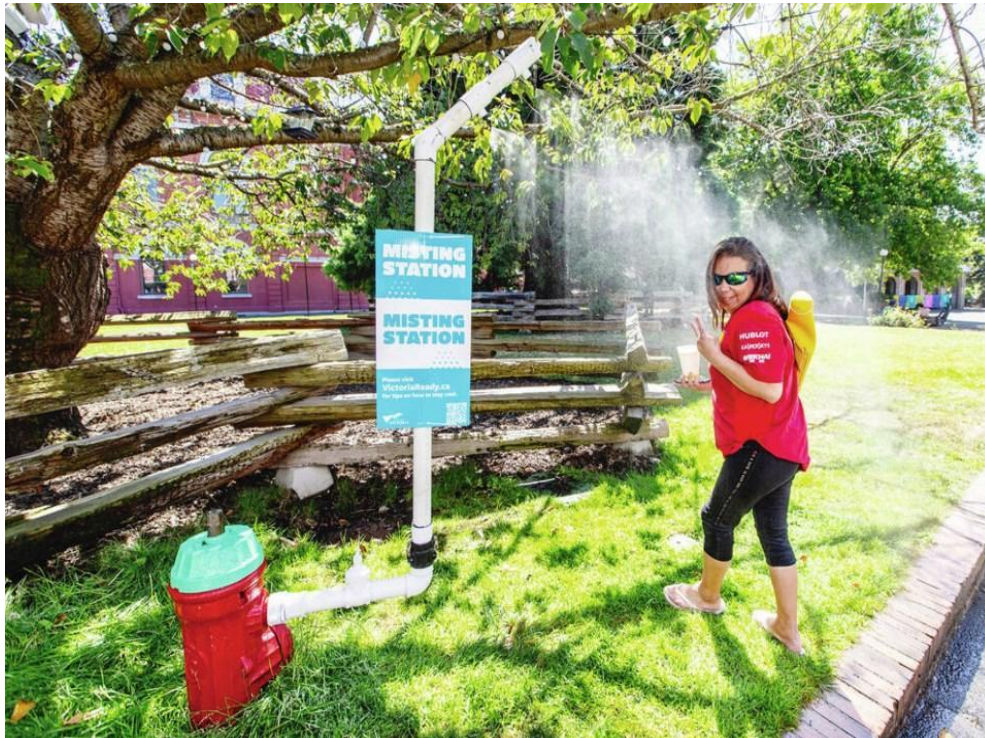
Figure 60: A misting station incorporated into a fire hydrant in Victoria, BC
