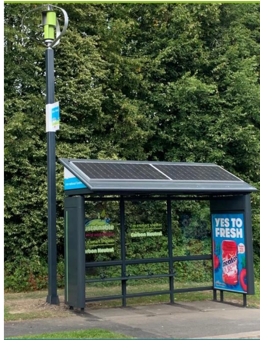
Figure 65: A wind and solar-powered transit shelter in Telford, UK
