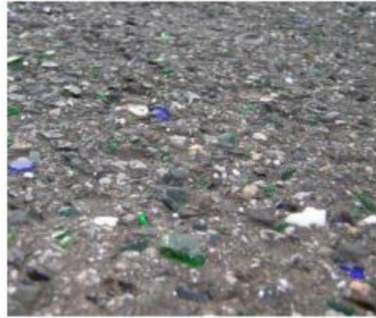
Fig. 5.8 Surface of a road constructed using glassphalt
