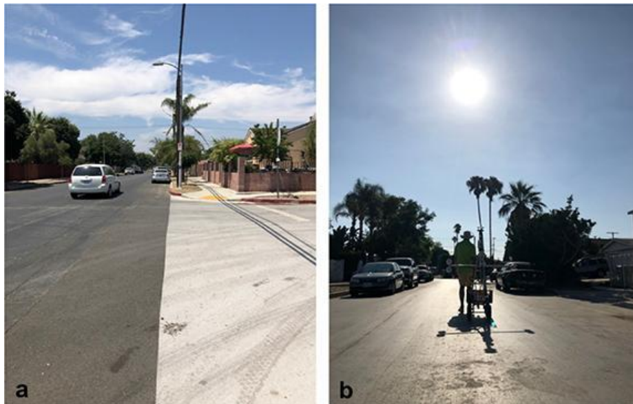
Figure 71: Solar reflective pavement coatings showing the difference between absorbent dark asphalt and light-coloured, reflective treatment
