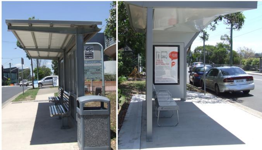
Figure 67: Original shelter shown beside the revamped, CAPS shelter
