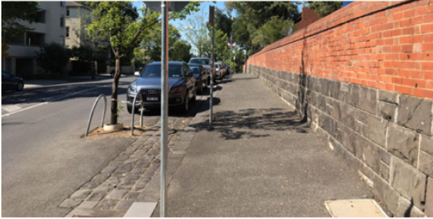
Original condition as a bitumen footpath (April 2017).
