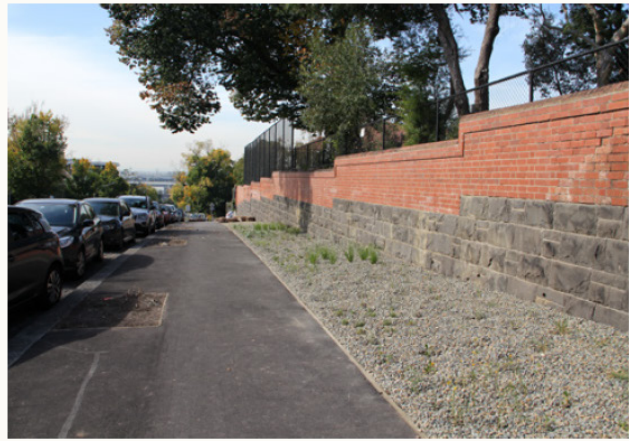
Plant installation (April 2018).
