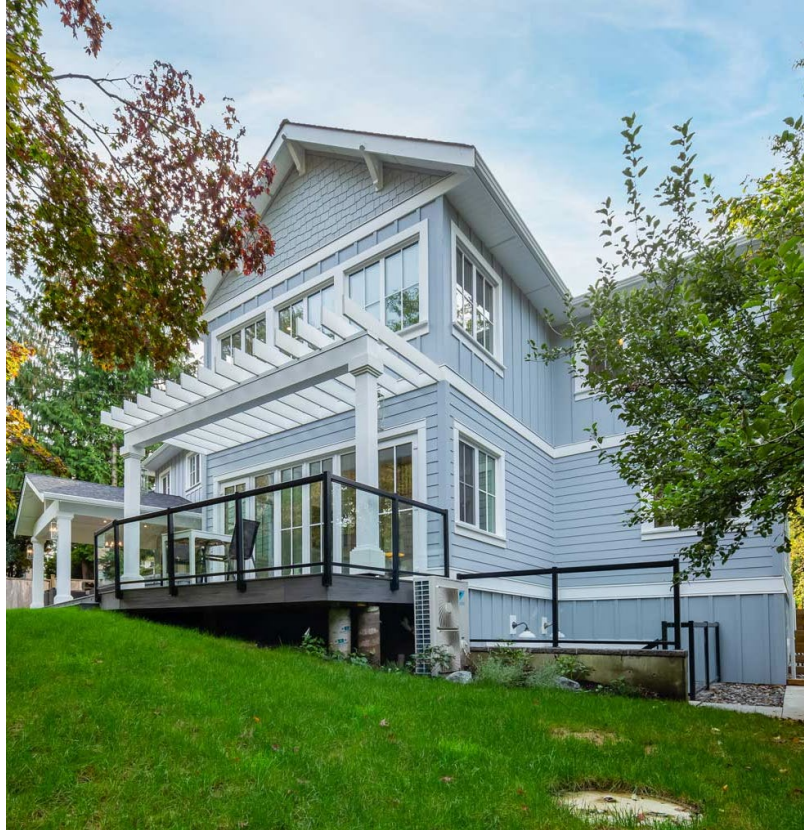
Figure 27: North-east façade of Burnaby NZER, exterior of the double height living room (Photo courtesy of Kemp Construction)
