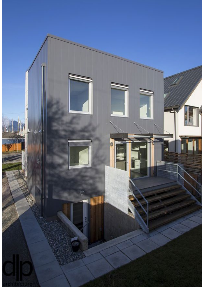
Figure 15: South Elevation of Casa Luca, more generous glazing on the facade allows for solar gains and daylighting, while exterior shading prevents overheating (Photo courtesy of DLP Architecture)
