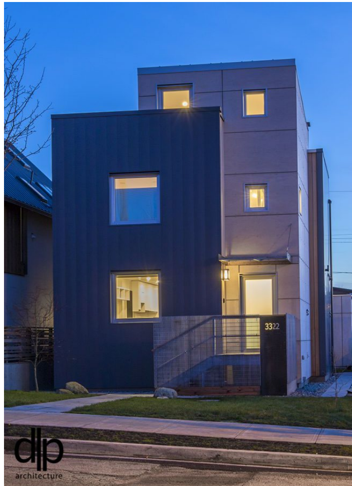
Figure 24: Front elevation of Casa Luca, glazing on the north façade is limited to prioritize solar gains on the south. (Photo courtesy of DLP Architecture)
