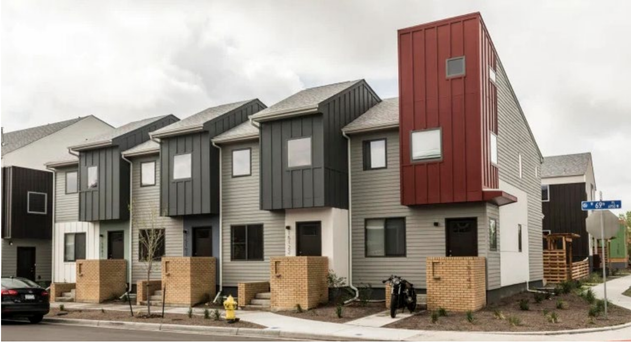
Figure 28: North elevation of the Geos Reihenhäuser (Photo courtesy of SUN Studio)
