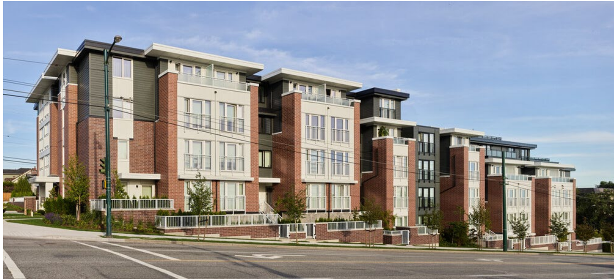
Figure 30: West facade of Spire Landing, stepped along the sloped site (Photo courtesy of Cornerstone Architecture)
