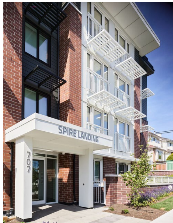
Figure 31: Sun shading devices of the south façade (Photo courtesy of Cornerstone Architecture)
