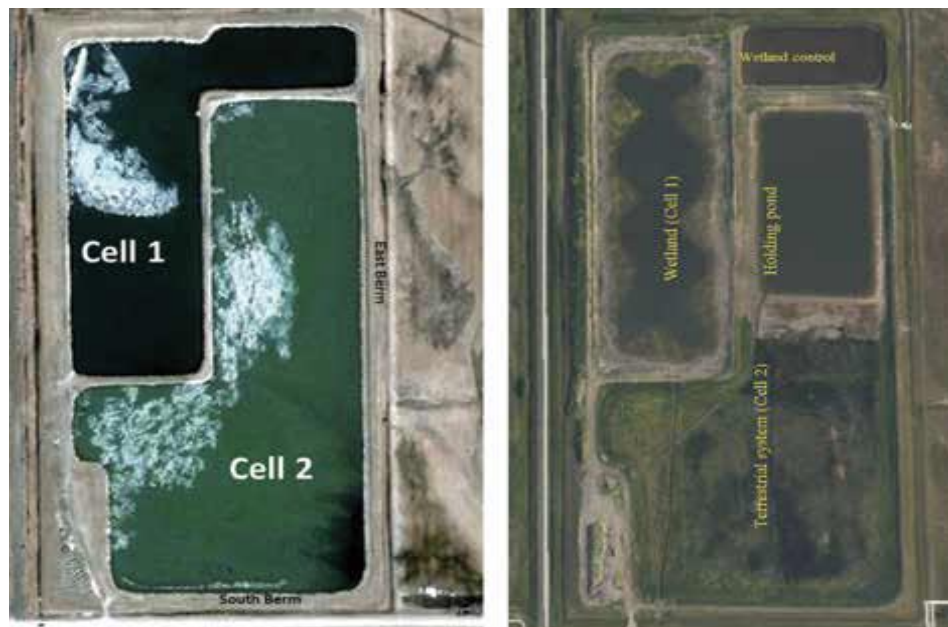
Figure 6 Former Niverville municipal wastewater treatment plant (left image) and current restored wetland layout (right image) (Jeke et al., 2016a).
