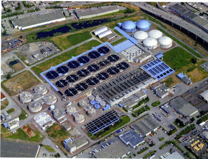
Figure 1. Annacis Island Wastewater Treatment Plant (AIWWTP) located at Delta, British Columbia, the largest wastewater treatment plant operated by Metro Vancouver, and treats wastewater from 14 municipalities in the Lower Mainland to safely discharge the same into the Fraser River 4 .
