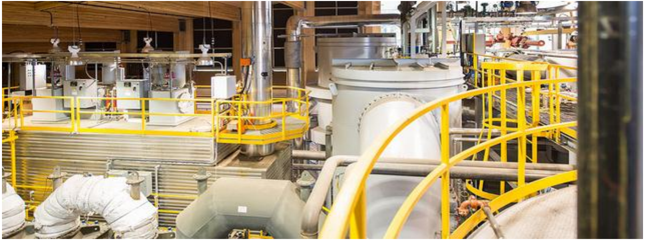
Bioenergy Research and Demonstration Facility Interior. Credit: Don Erhardt
