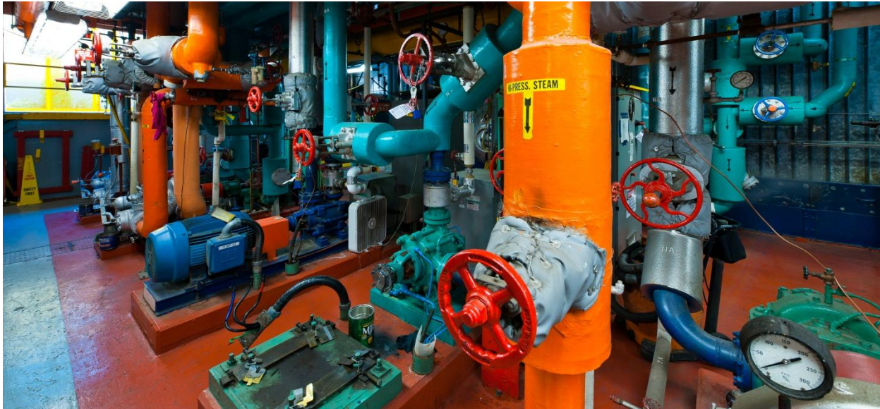
Converting UBC's district heating system from steam to hot water will reduce emissions by 22 per cent. Credit: Don Erhardt
