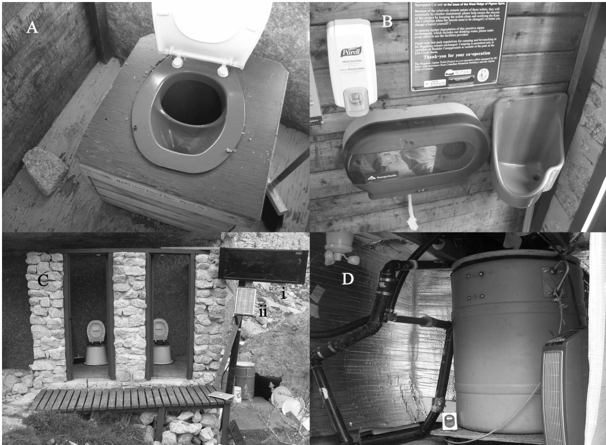
Fig. 2.1 Alternative toilet waste management treatments at Kain Hut, Bugaboo Park, B.C. Canada. A) Urine diversion toilet seat. B) Urinal with 1” braided drain pipe to collection barrel. C) Lower toilets with UD12V solar hot air panel (i) above a 5W PV panel (ii). D) Upper Kain Hut toilet insulated basement, 110V heater, and 110CFM exhaust fan positioned around a 200L plastic barrel with double garbage bags to collect solids.
