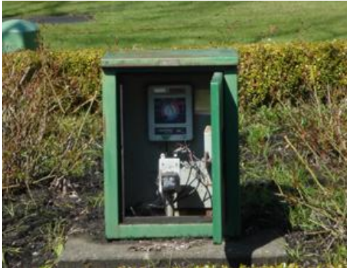
Figure 6: Electrically controlled and powered sprinkler system
