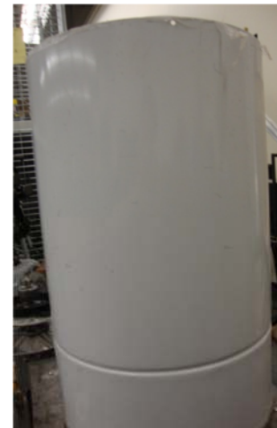
Figure 34: Spinner Casing to be cut
