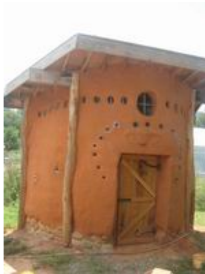
Figure 2: Cob Recycling Office and Shed
