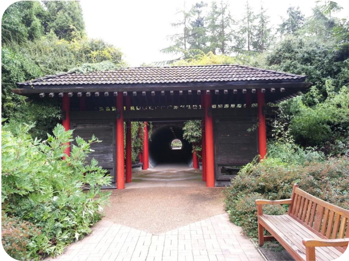
Figure 4: Existing Tunnel; the Moon Gate
