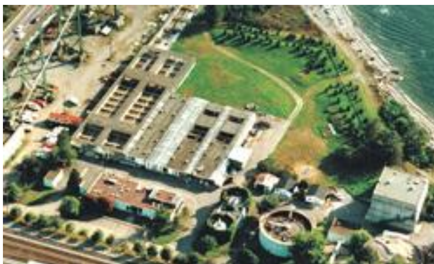
Figure 2: Lions Gate Wastewater Treatment Plant
