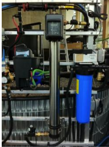
Figure 5: The UV Filter at CIRS Building ( EcoTek Slides, 2012 ).
