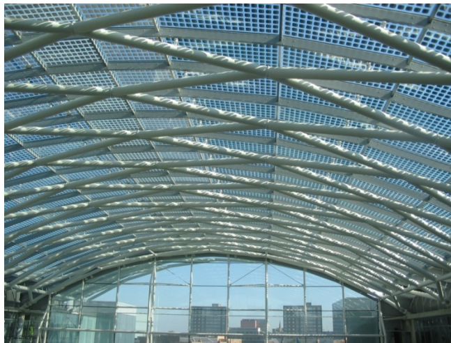
Figure 4: PV cells integrated into the design of a building Source: www.pv-tech.org
