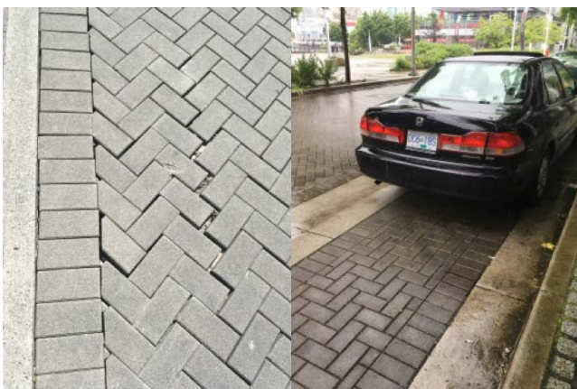
Example of conventional pavers spreading due to the inverted crown design (left) and permeable pavers performing successfully during a rainfall event (right).
