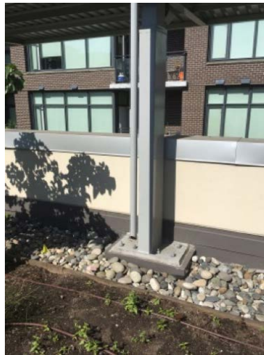
Rainwater harvesting in one Olympic village building: A collection spout empties rainwater from a building roof and podium onto a gravel bed, which then is connected to the rainwater cistern in the building’s basement
