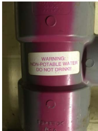
Purple pipes labelled as containing non-potable water
