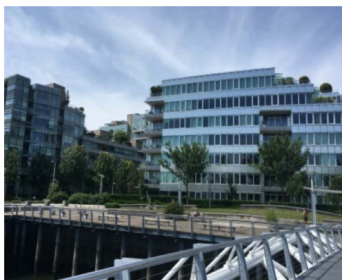
Section of the sea wall in front of Olympic Village.
