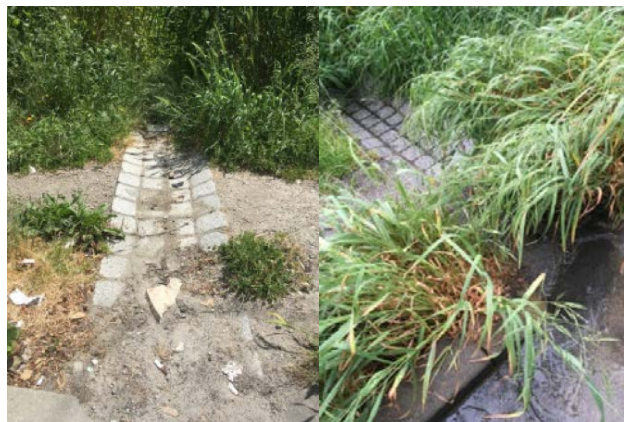
Clogged bioswale inlets on a dry day (left) and a wet day (right) (June 2017).
