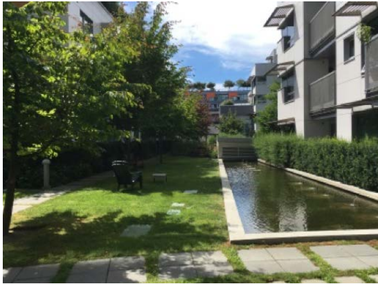
Intensive green roof and rainwater water feature
