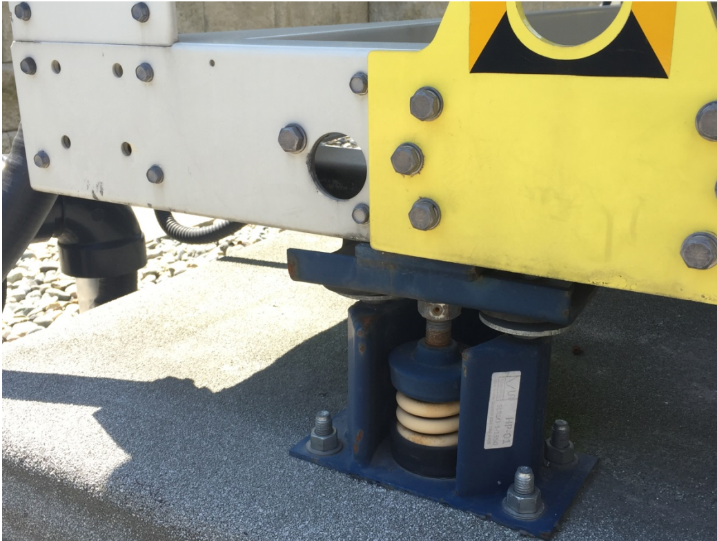
View of vibration isolation air shocks underneath Aermec NRP 1800 unit.
