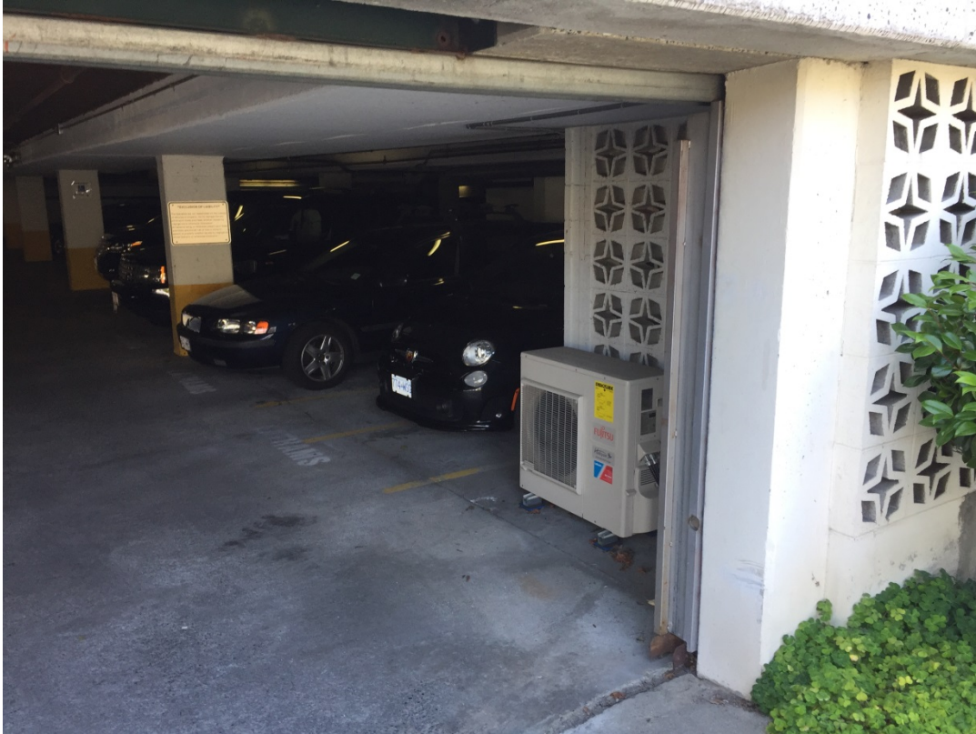
Example of single heat pump unit located in ground-floor parking garage.
